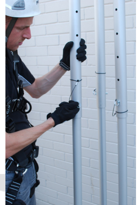
Fig. 3 Lock individual legs with pins.
